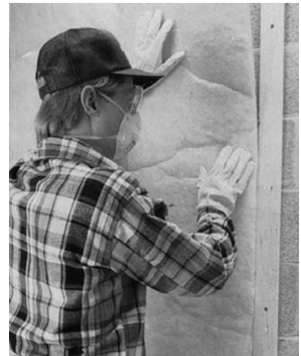
MASONRY WALL INSULATION
