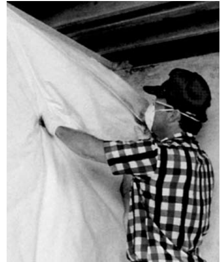
BASEMENT WALL INSULATION
